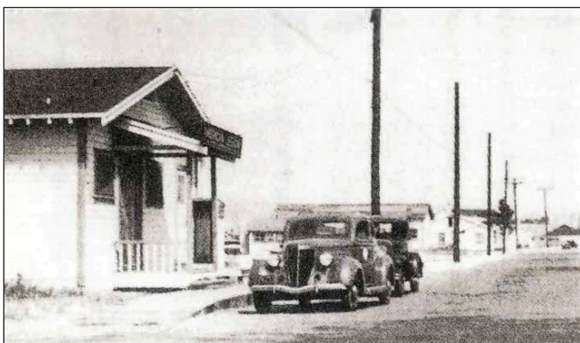
Original Post 291 Hut on 10th St. looking East (Photo courtesy Ken Taylor)
