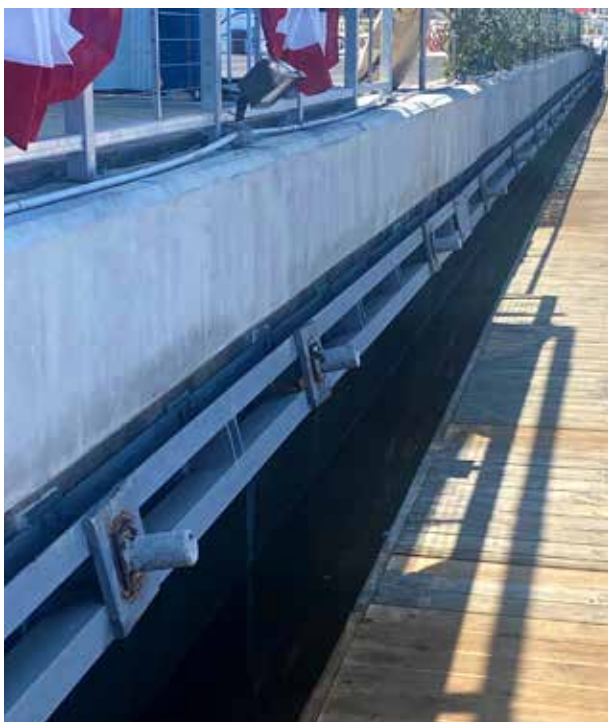
Seawall (left) braces added by the City of Newport Beach
